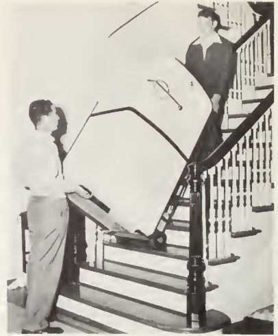
17-9. Correct method of handling a refrigerator on stairs. Note how the roller tread assists over stair treads. (Stevens Appliance Truck Co.)
